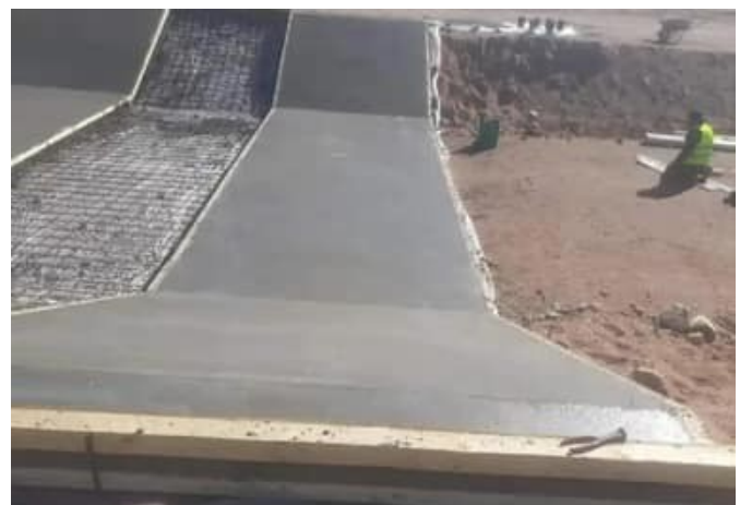
Channel side finishing
