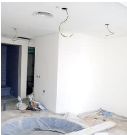
Room after finishing
