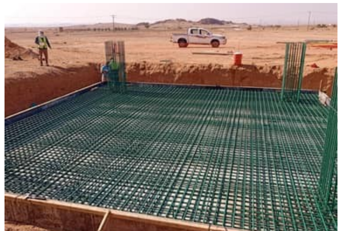
Tower foundation reinforcement
