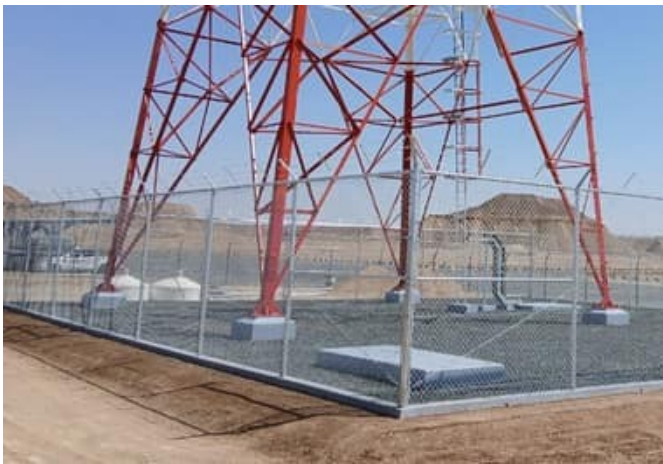
Tower compound fencing
