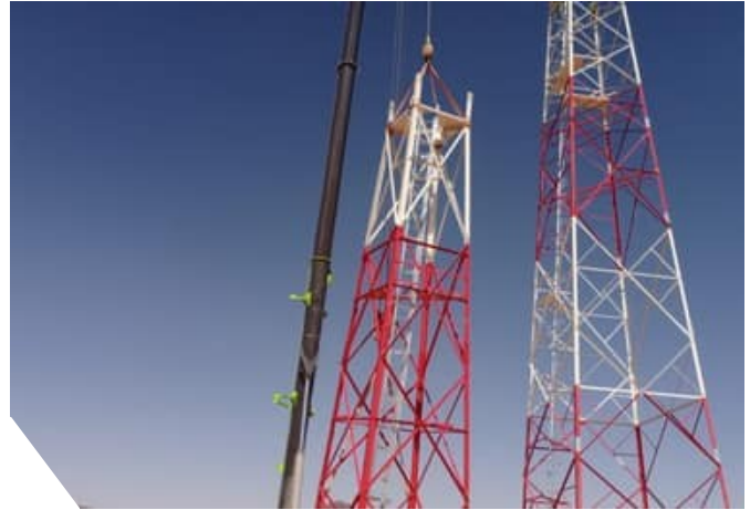
Crane erection of two towers
