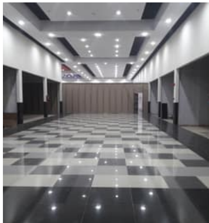
Hall after finishing and lighting
