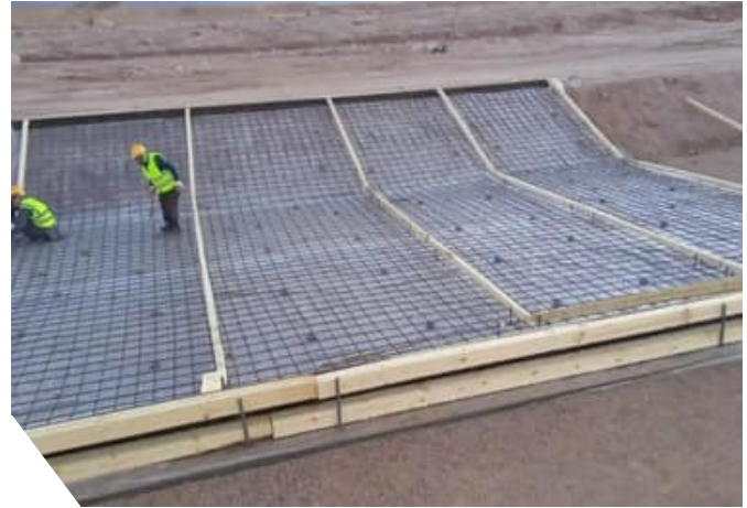
Placing reinforcement mesh
