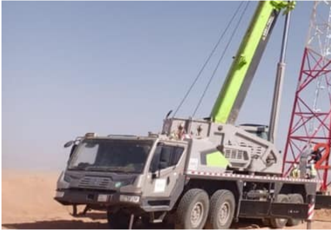
Lifting tower sections
